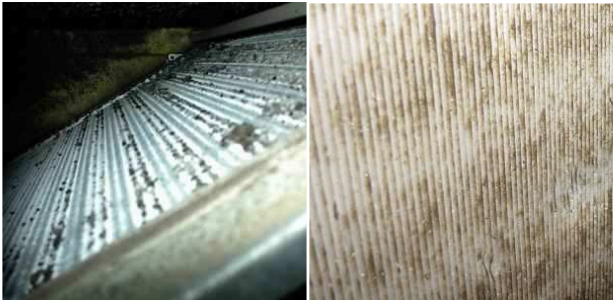
Fungal Biofilm Growth on a Residential (Left) and Commercial (Right) Cooling Coil
