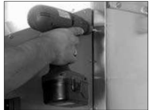
Figure 2.3c - Install unit using all supplied fastening hardware.
