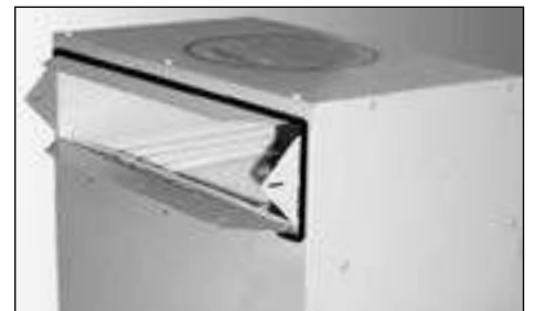
Figure 2.2j - Bend tabs outward 90 degrees.
