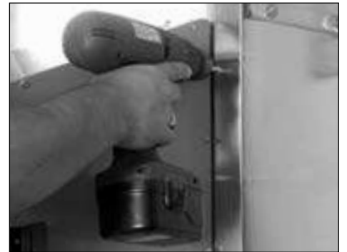
Figure 2.3c - Install unit using all supplied fastening hardware.
