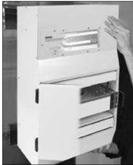
Figure 2.3a - Align unit into place.
