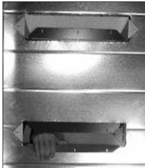
Figure 2.3b - Unfold the ducting flairs to sandwich the return air plenum between the ducting flair and the filtration unit.
