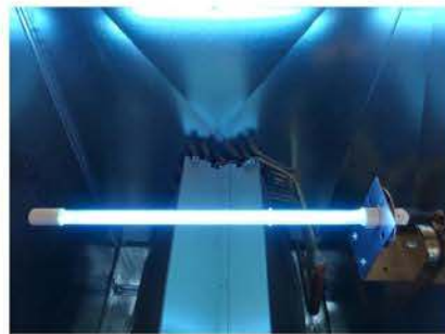
Low voltage 24VAC ballast w/ Lamp and Ballast Monitoring Electronics
