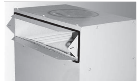
Figure 2.2j - Bend tabs outward 90 degrees.
