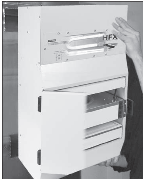
Figure 2.3a - Align unit into place.
