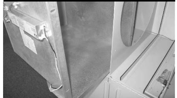
Adhere the included foam gasket (incl. in the Lamp box) to the porcelain end-cap with the 4 pins.
