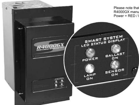
Please note that the R4000GX ballast was changed in 2009. Those R4000GX manufactured prior to 2009 had the following LED colors: Power = RED / Ballast = GREEN / Sensor = AMBER / Lamp = BLUE
