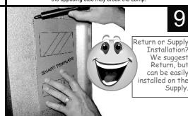
Draw around the 'Smart Template' outlining where the Purifier will be installed
