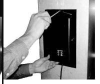
Use the self-taping screws (included) to mount the purifier to the duct. Just plug into an electrical socket and turn on the red toggle switch
